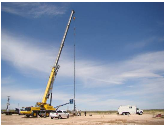
Figure 27: Well Site during workover
