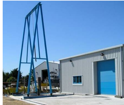
Figure 8 Gantry, test well and works
