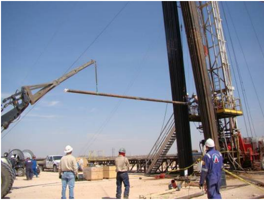
Figure 20: BHA Being Installed
