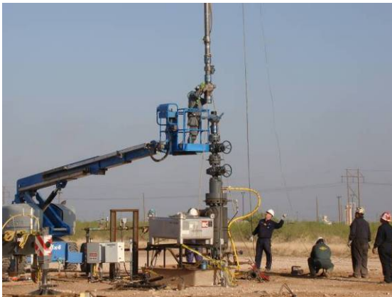
Figure 26: Lubricator attaching to Wellhead
