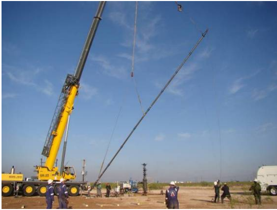
Figure 25: Crane Lifting Lubricator
