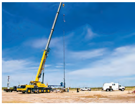
Fig. 7. ALC crane and lubricator during Rigless ESP installation.
